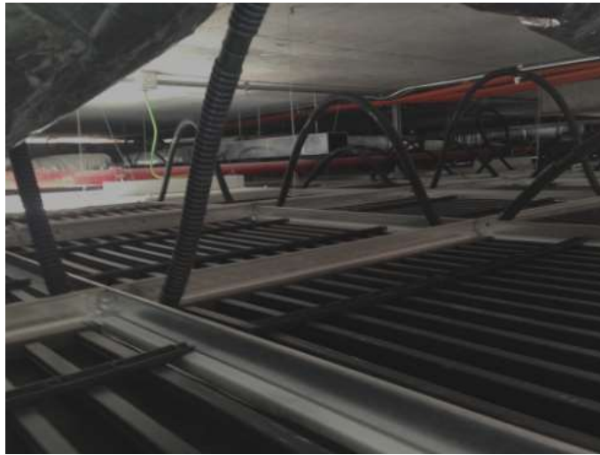
Figura 3.17. Cielo radiante ( https://pansogal.com/ )
